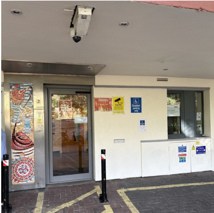
The entrance to the building.
